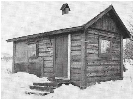
A typical sauna building
