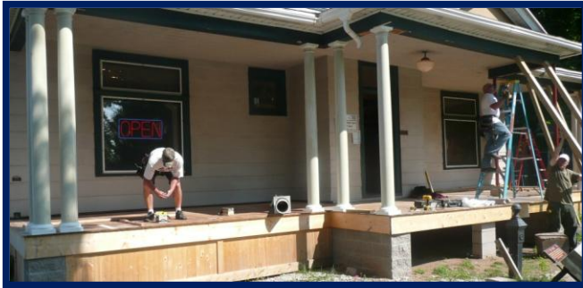
Repairs finally authorized, work begins – August 2013
